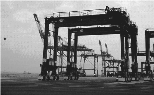
Figure P1.11 Photo of a rubber-tired gantry crane.
